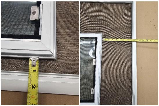
**Step 8:** Once you have measured the pet screen out and assured it is level, apply painters tape to keep it from moving. This may take quite a bit on larger screens. The goal is to flip the whole unit over without displacing the pet screen. Once it is flipped over to expose where you would like to apply the spline, re-measure to assure the pet screen is still in the place you desire.
